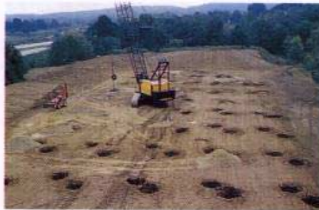
Collapsing sinkholes/soil voids at column locations, Valley Forge, Pennsylvania
