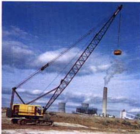
Loose sands at power plant near Jacksonville, FL improving to 25 ft.
