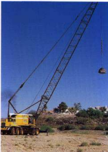
Retail Center next to "Ping" residence, Phoenix AZ
