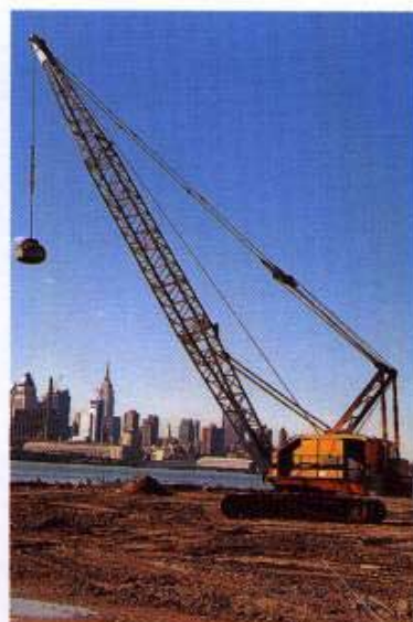
Rubble fill site, New York City
