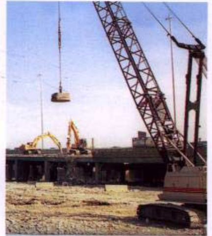
Reconstruction of Stevenson Expressway, Chicago, IL
